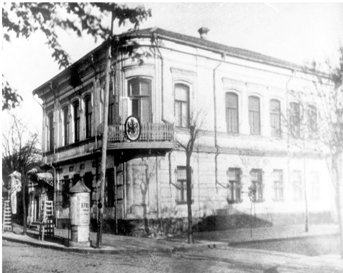
62. The building of the plant management
