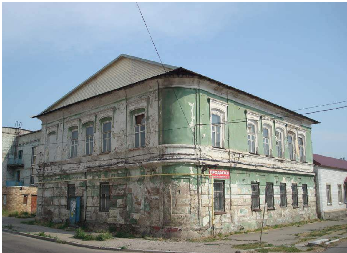
63. The former building of the plant management and the British Vice-Consulate
